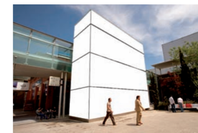
VAP VINILO ASCENSOR PATIO CENTRAL DOS FRENTES VINYL ELEVATOR CENTRAL COURT TWO FRONTS 10,40 x 9,85 + 3,45 x 9,85 m
